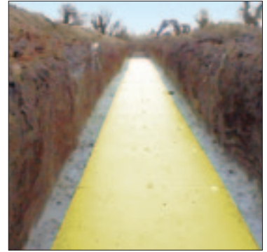
Milled protection sheets for gas pipes
